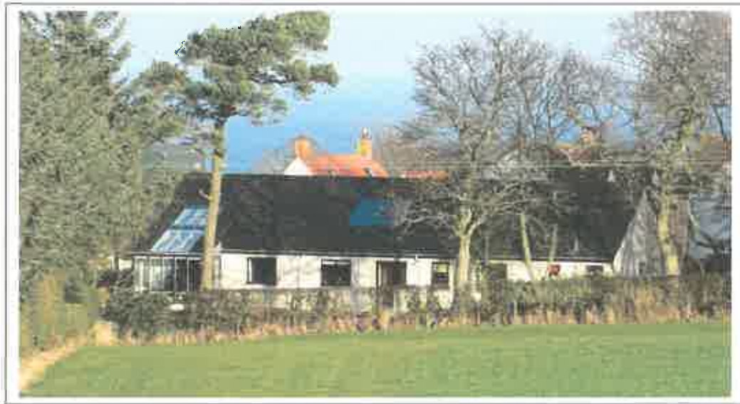
Site adjacent to building group would destroy the privacy of the adjacent Dwellinghouse and would struggle to meet with the requirements of Policy HD3
