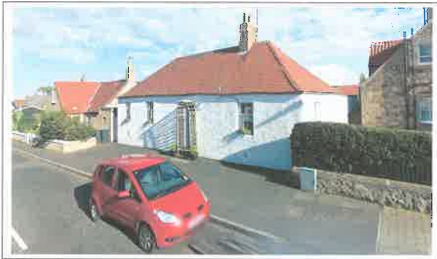
Typical house construction in Cockburnspath with stone and rendered walls and pitched pantiled Rosemary tile and slate roof coverings
