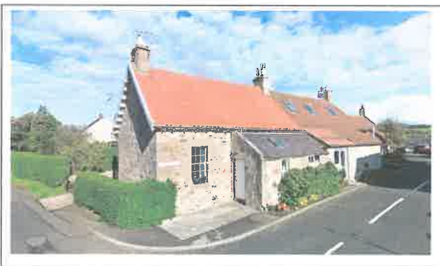
Typical house construction in Cockburnspath with stone and rendered walls and pitched pantiled Rosemary tile and slate roof coverings
